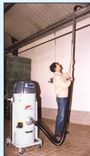
External pipe cleaning
